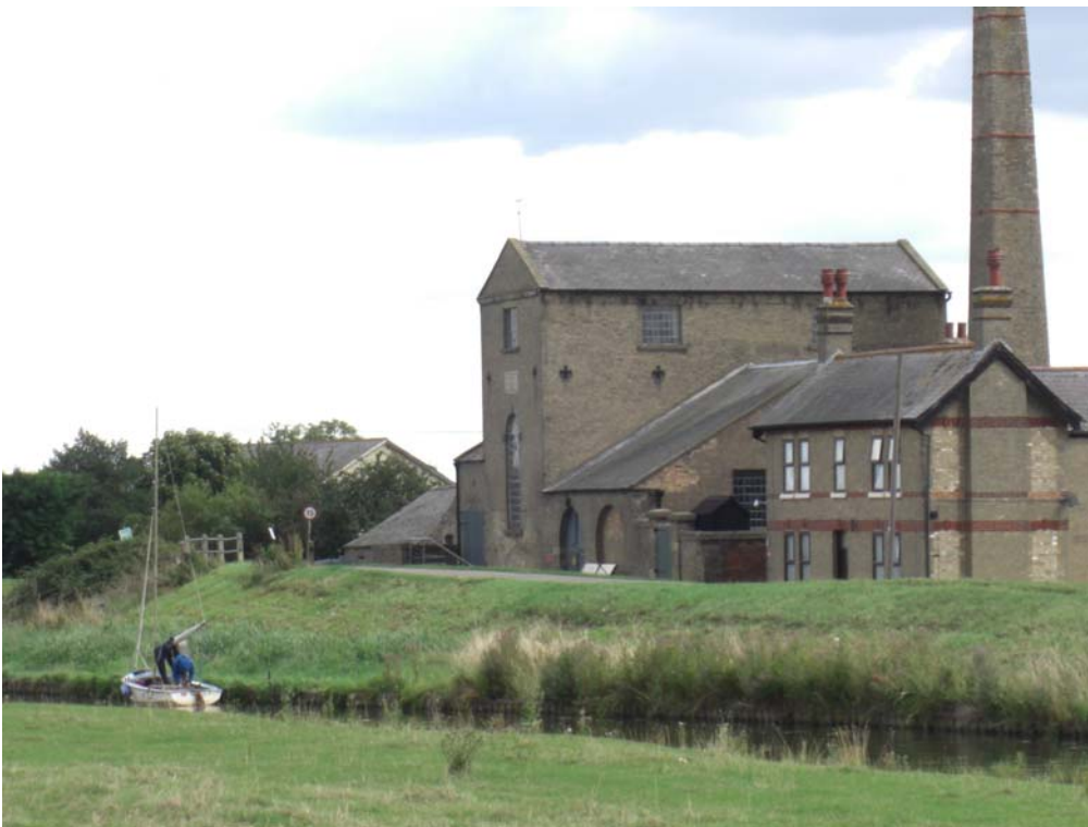
Streatham Pumping Station
